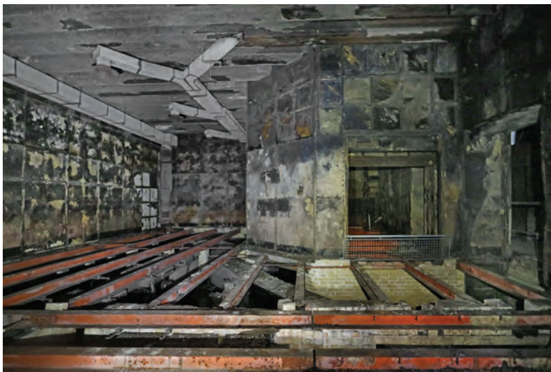
The Track Telling room with plotting room in the corner
